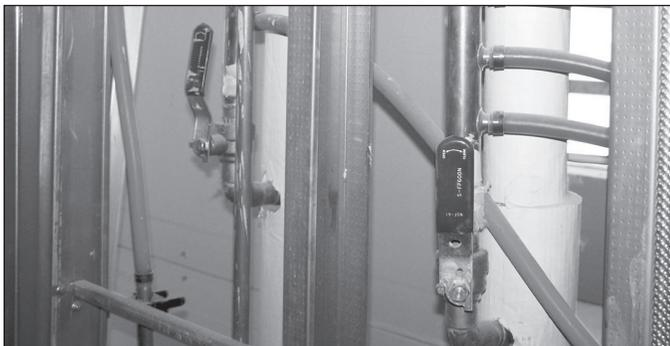
Zurn PEX tubing connected to copper manifolds using copper crimp rings.
