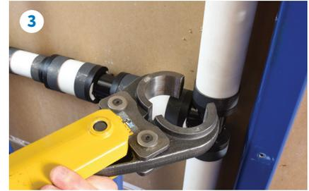
3 Open jaws of crimp tool (QCRBTKIT56-14V power tool shown), and place over properly aligned QickCap crimp ring.
