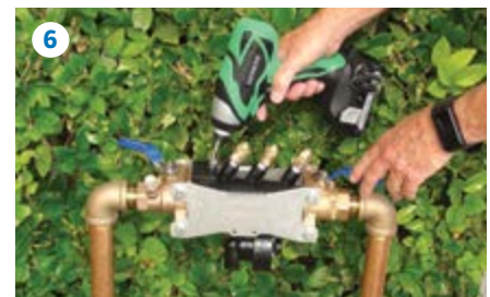
In spring, attach hose and flush the line to remove any debris. Remove Blow-Out Accessory, reinstall EZSwap, and commission the backflow to start-up the system.
