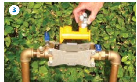
Insert and install the Blow-Out Accessory.
