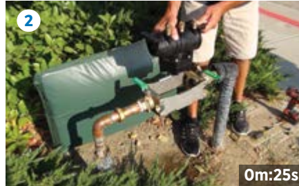
Un-bolt or un-screw and remove EZSwap Pressure Vessel.
