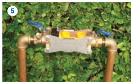
Remove air hose and leave Blow-Out Accessory installed for the winter as a visual indicator. Leave shut-off valves in the half open and half closed position to prevent freeze damage.
