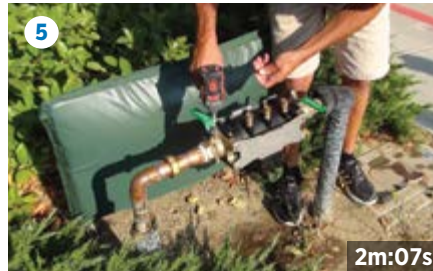
Remove Flush Fitting Tool and reinstall EZSwap Pressure Vessel.
