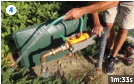
Attach hose to Flush Fitting Tool and turn on inlet ball valve. Direct water to landscaping or safe drain and flush until clear.
