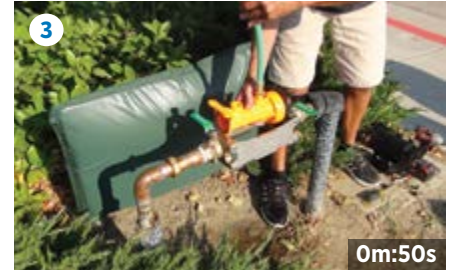
Drop in and install Flush Fitting Tool.
