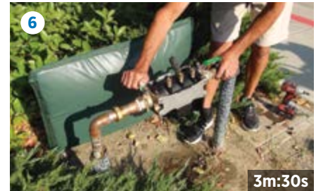
Commission the backflow and start up system.
