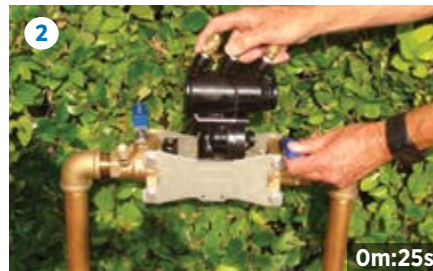
Unscrew and remove wedge, or un-bolt. Remove EZSwap™ from body. Store EZSwap indoors for the winter.
