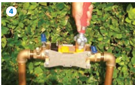
Attach air hose to Blow-Out Accessory and turn on compressor. Manually blow-out each zone to evacuate water.
