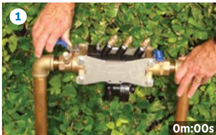
Valve is installed in-line. Turn shut-off valves to shut down system. Open test cocks to relieve pressure.
