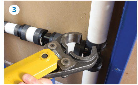
3 Open jaws of crimp tool (QCRBTKIT56-14V power tool shown), and place over properly aligned QickCap crimp ring.
