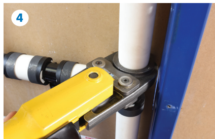
4 Crimp the ring to create a permanent, leak-free connection.
