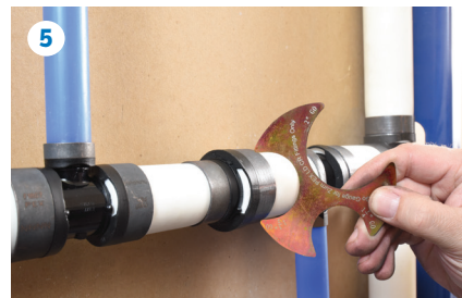
5 Use gauge (large diameter Go-Go Gauge, QGA678CR shown) to verify that a secure crimp has been made.
