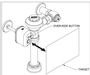
**Step 4-** Check actuator to ensure sensor is working. Hold manila folder at edge of the toilet for 10 seconds. Remove and actuator should flush valve.
