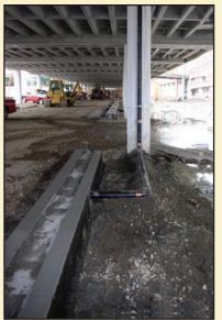
Trench drain from the upper deck was tied into the lower with 4-inch cast iron soil pipe fitted through the trench drain side wall.
