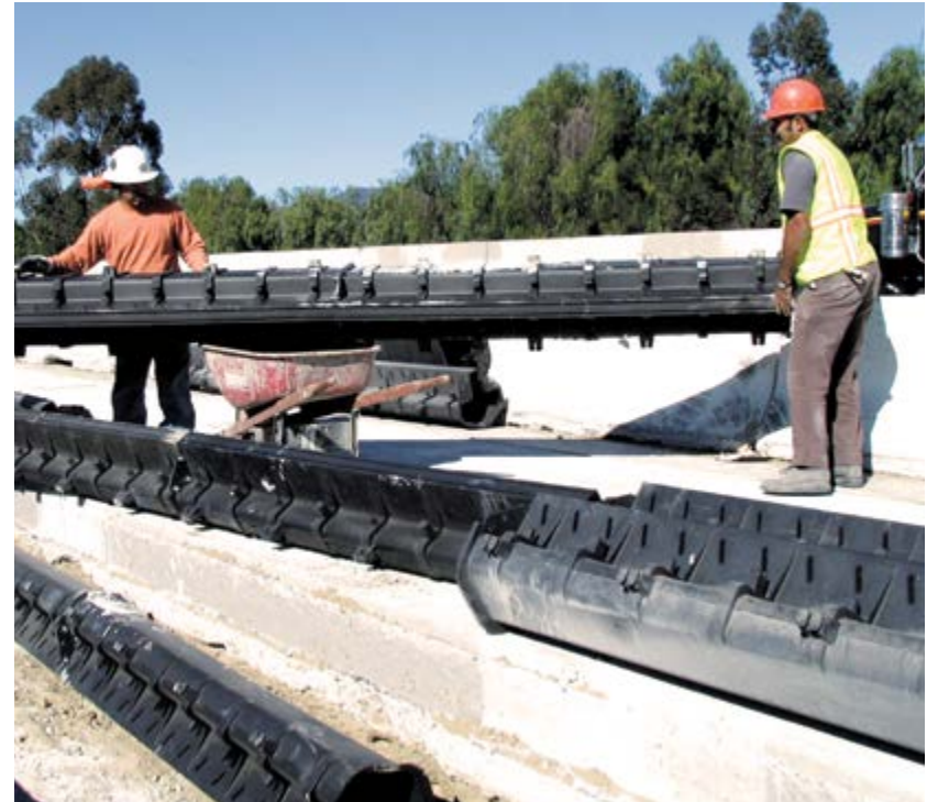
Two workers (and no equipment) easily lift and install our Z888 Hi-Cap® trench drain.
