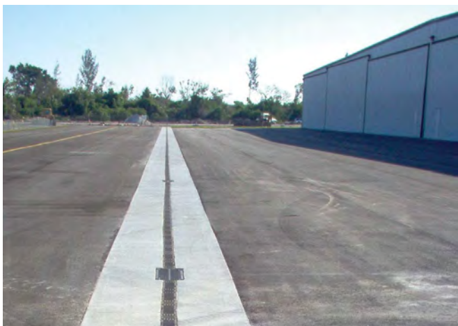
Airport Trench Drain
