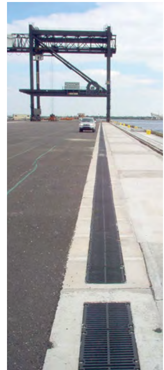
Port Trench Drain
