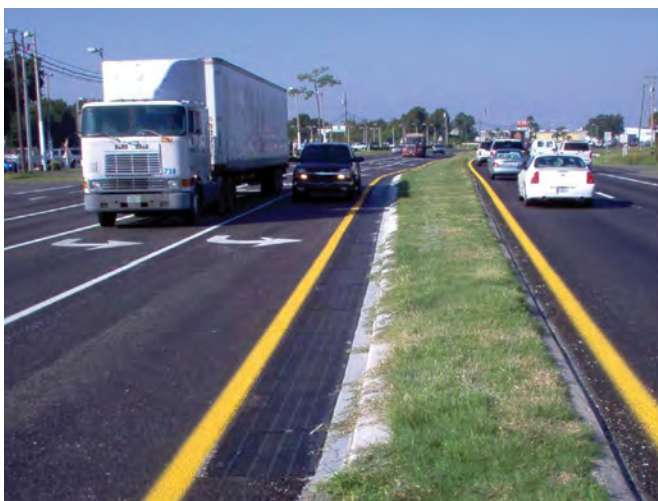
Median Trench Drain
