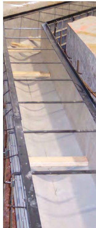
Airport Trench Drain
