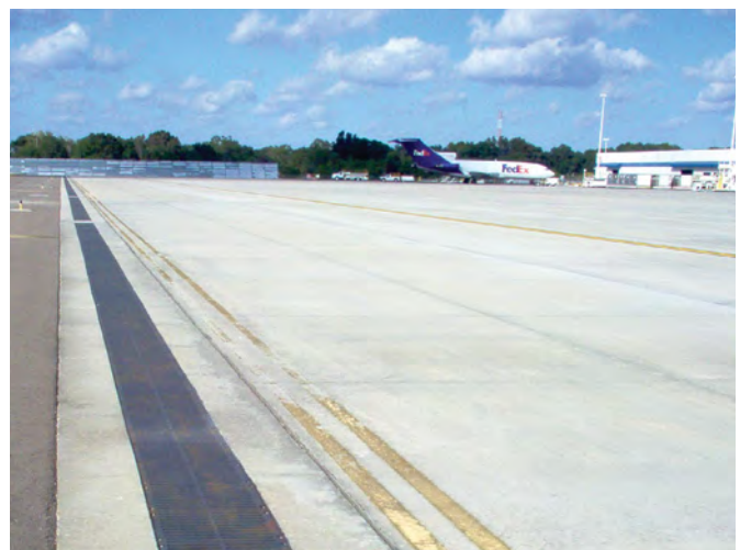
Airport Trench Drain
